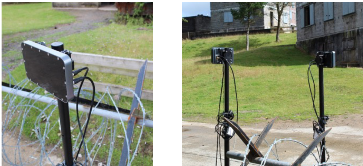
Figure 30: SDR ground surveillance radar, installation of the system for the demo.
